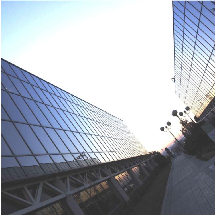
Corporate Headquarters and R&D Centre and Technological Demonstration of Invensys Rail Dimetronic at Parque Empresarial San Fernando (San Fernando de Henares)
