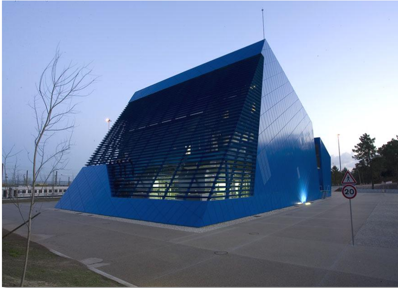
REFER's Operational Control Centre at Porto (Portugal)
